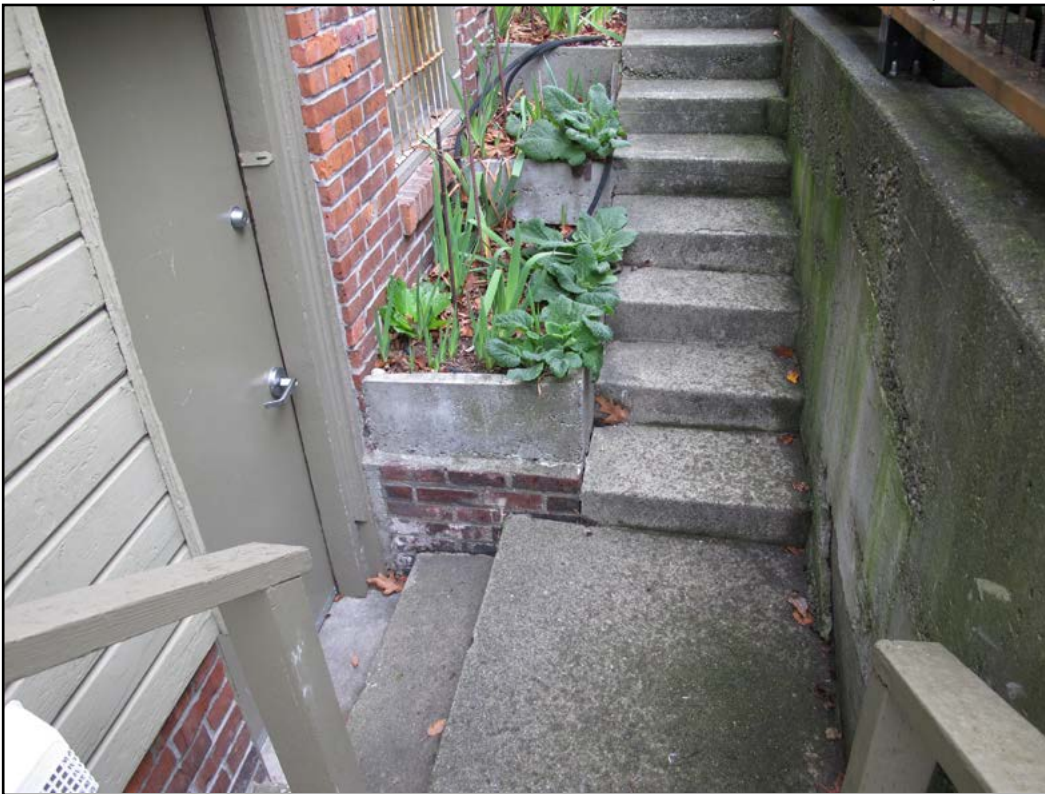
Figure 40 • Former parsonage building, stairs and door to eastern basement, eastern façade
