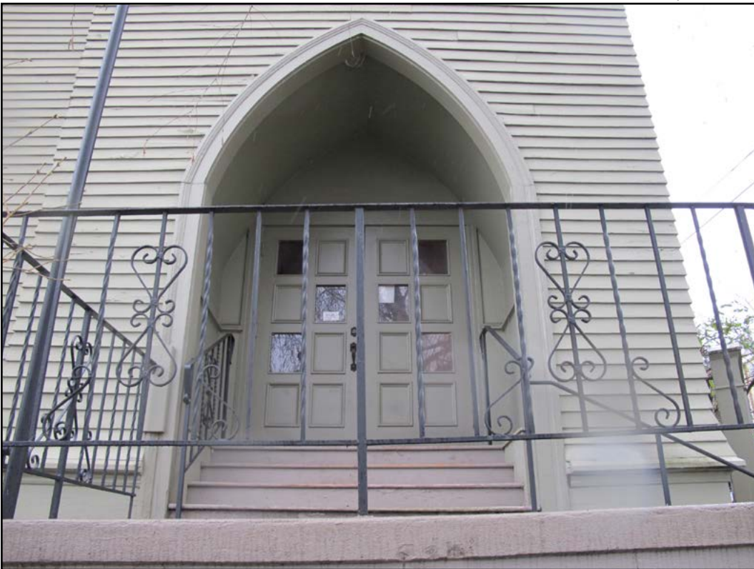
Figure 13 • Former church building, entry on eastern façade
