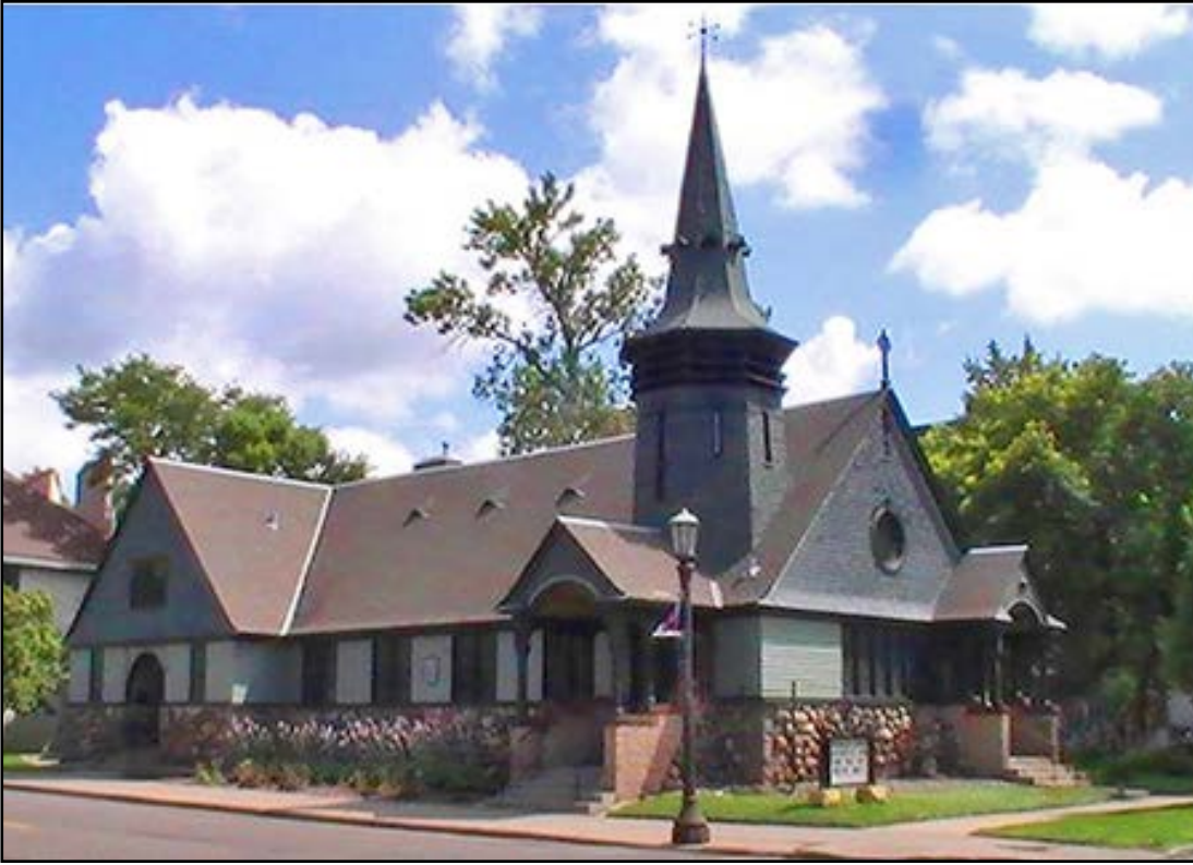
Figure 71 • Virginia Street Swedenborgian Church, Saint Paul, MN (1886, Cass Gilbert, Gilbert & Taylor, National Register)
