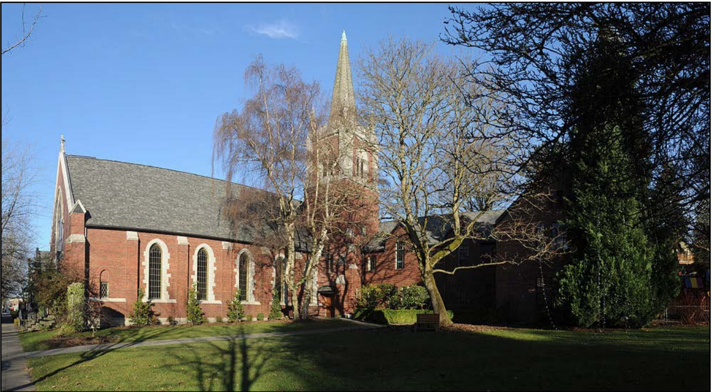
Figure 52 • Bethany Presbyterian Church, 1818 Queen Anne Avenue N (1929-30, Charles Hay, City of Seattle Landmark)
