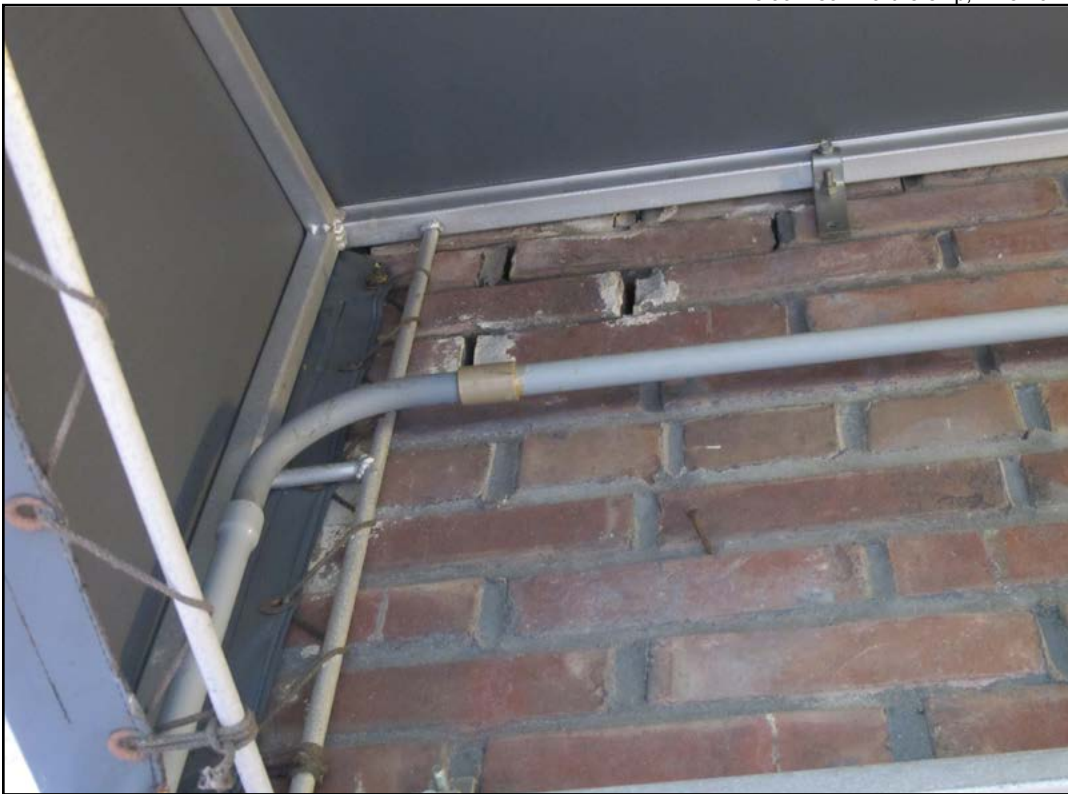
Figure 31 • Exterior view of damaged brick foundation near main entrance.
