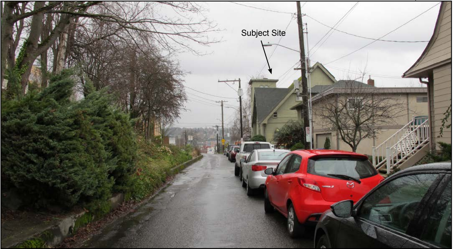
Figure 4 • View A - Viewing east on Valley Street
