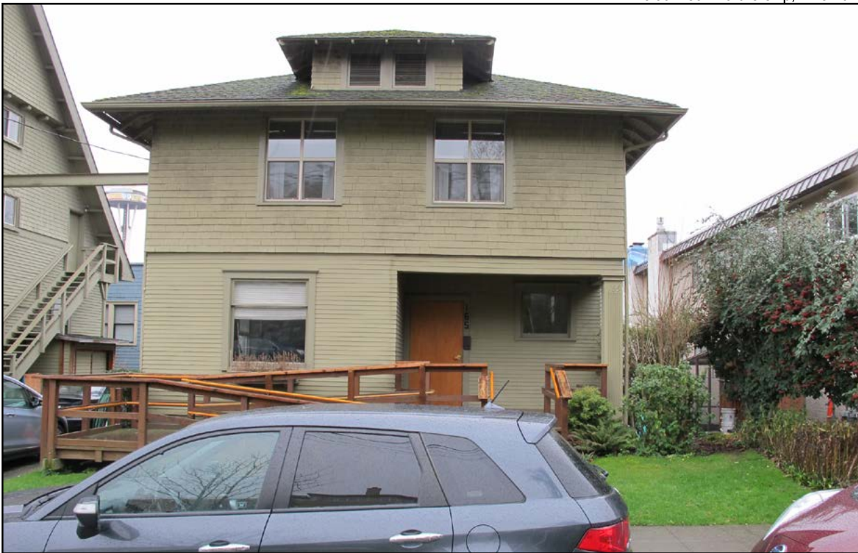
Figure 33 • Former parsonage building, northern façade
