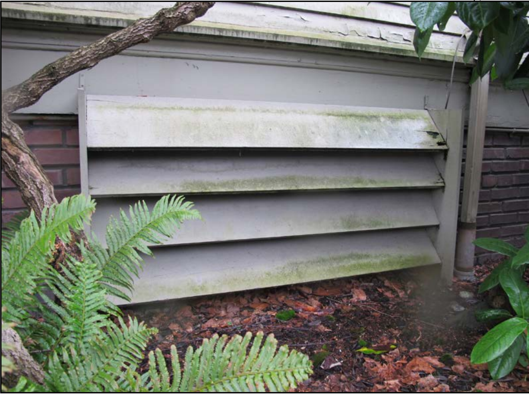
Figure 16 • Former church building, basement vent at northern façade
