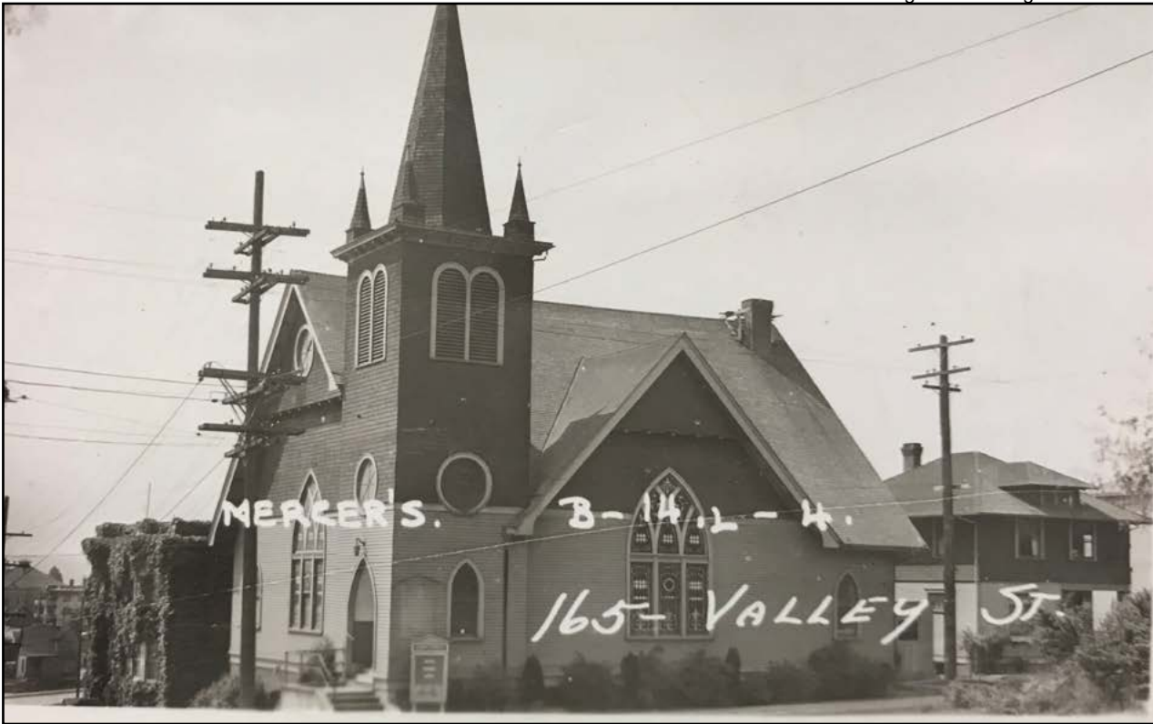
Figure 61 • Former church building, Tax Assessor Photo, 1937
