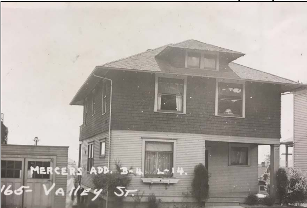
Figure 62 • Former parsonage building, Tax Assessor Photo, 1937
