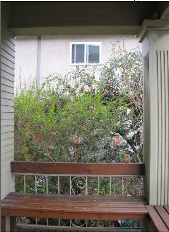
Figure 35 • Former parsonage building, porch at entry, northern façade
