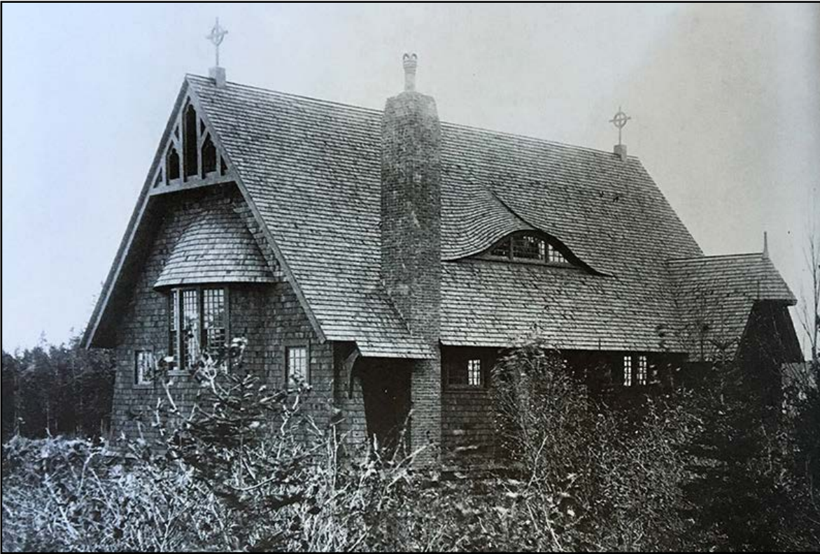
Figure 65 • St. Jude's Episcopal Church, Seal Harbor, ME (1887, William Ralph Emerson, National Register)
