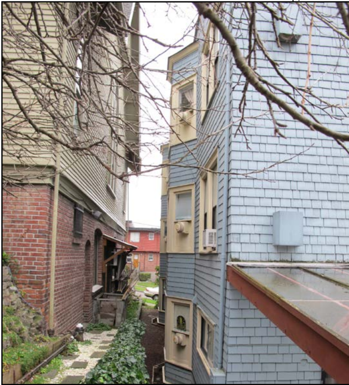
Figure 19 • Former church building, southern façade viewing from west
