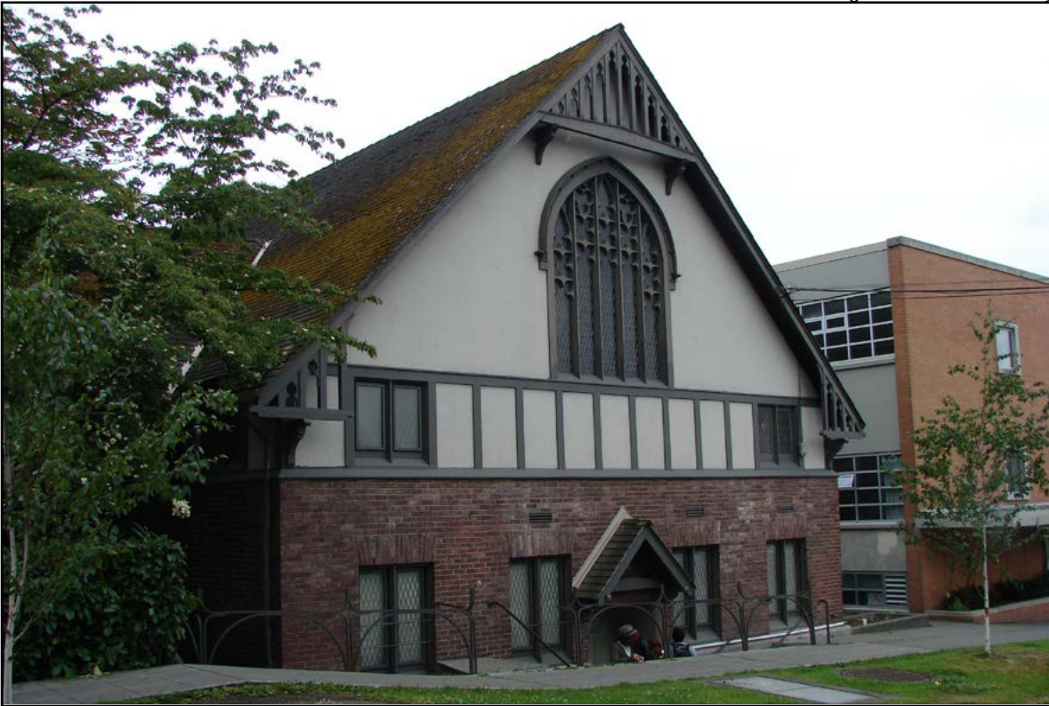
Figure 89 • University Presbyterian Church, 4555 16th Avenue N (1915, Ellsworth Storey, City of Seattle Landmark)
