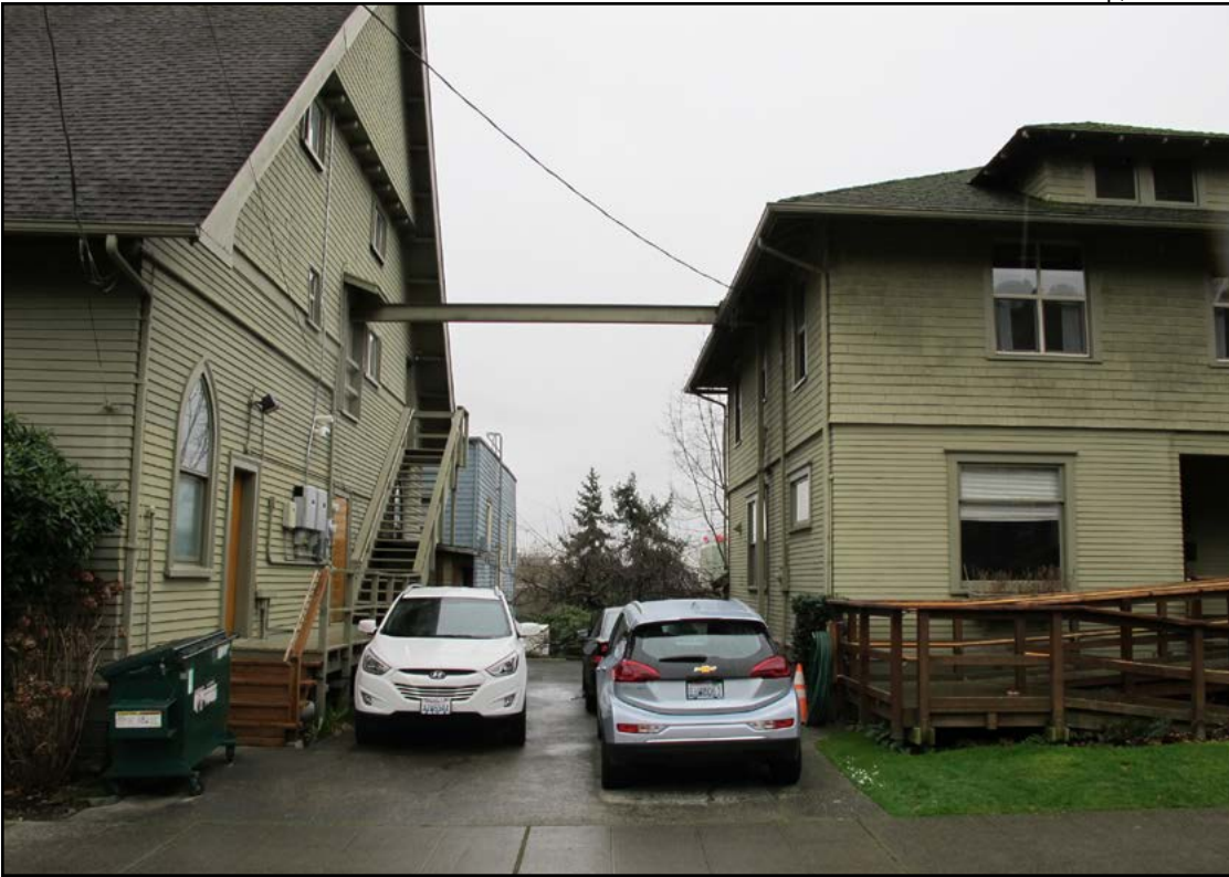
Figure 34 • Steel beam connecting former church and parsonage buildings
