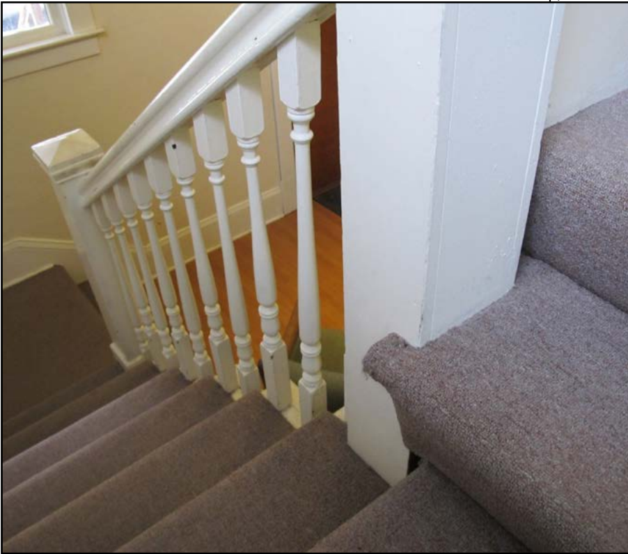
Figure 44 • Former parsonage building, second floor stairs
