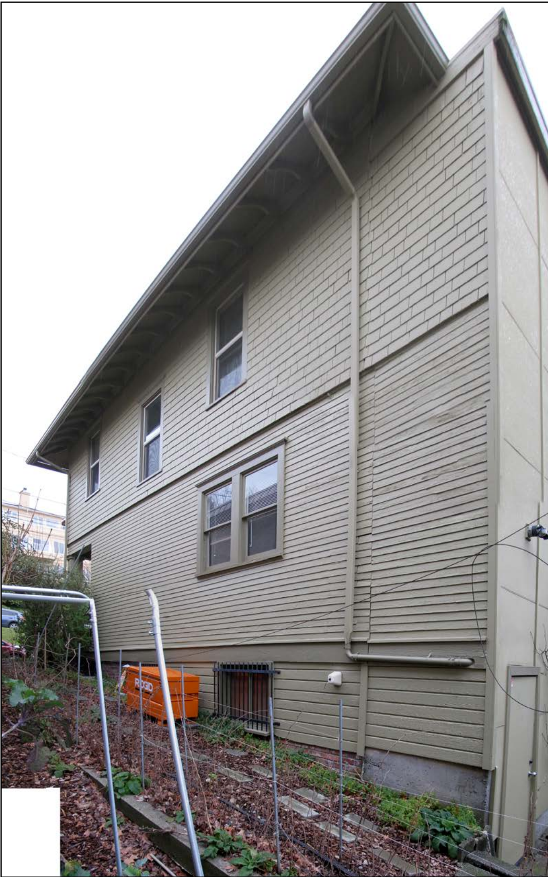
Figure 36 • Former parsonage building, western façade
