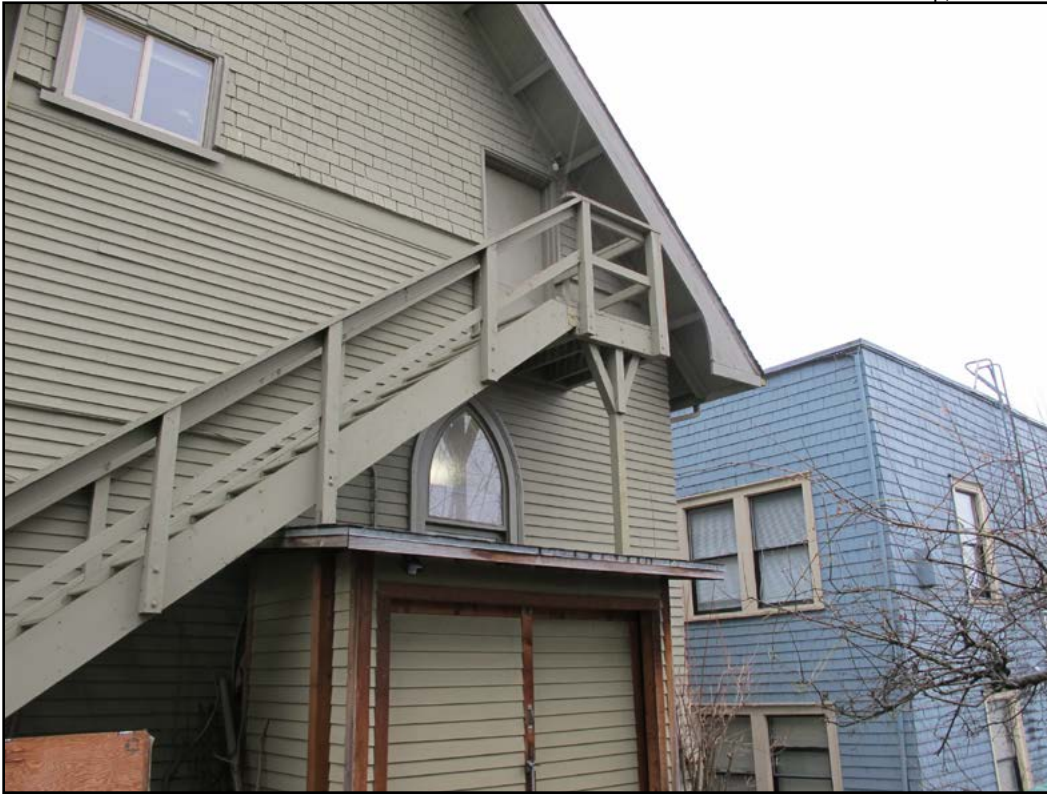
Figure 18 • Former church building, stair and storage shed, western façade
