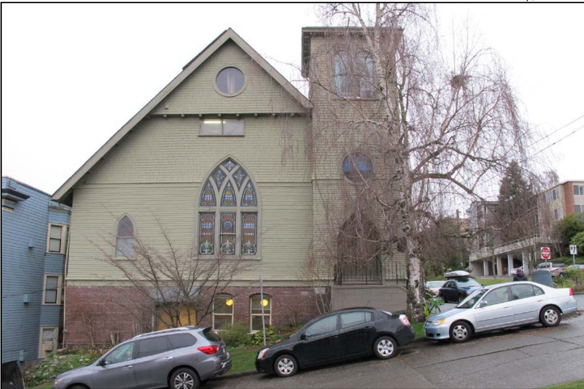
Figure 11 • Former church building, eastern façade
