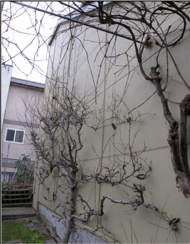
Figure 38 • Former parsonage building, detail at southern façade
