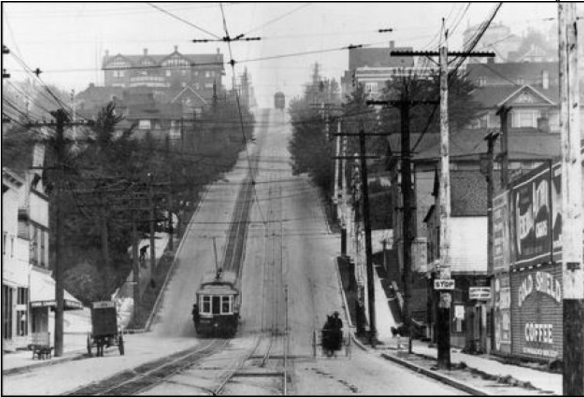
Figure 49 • Queen Anne Avenue Counterbalance, built 1905
