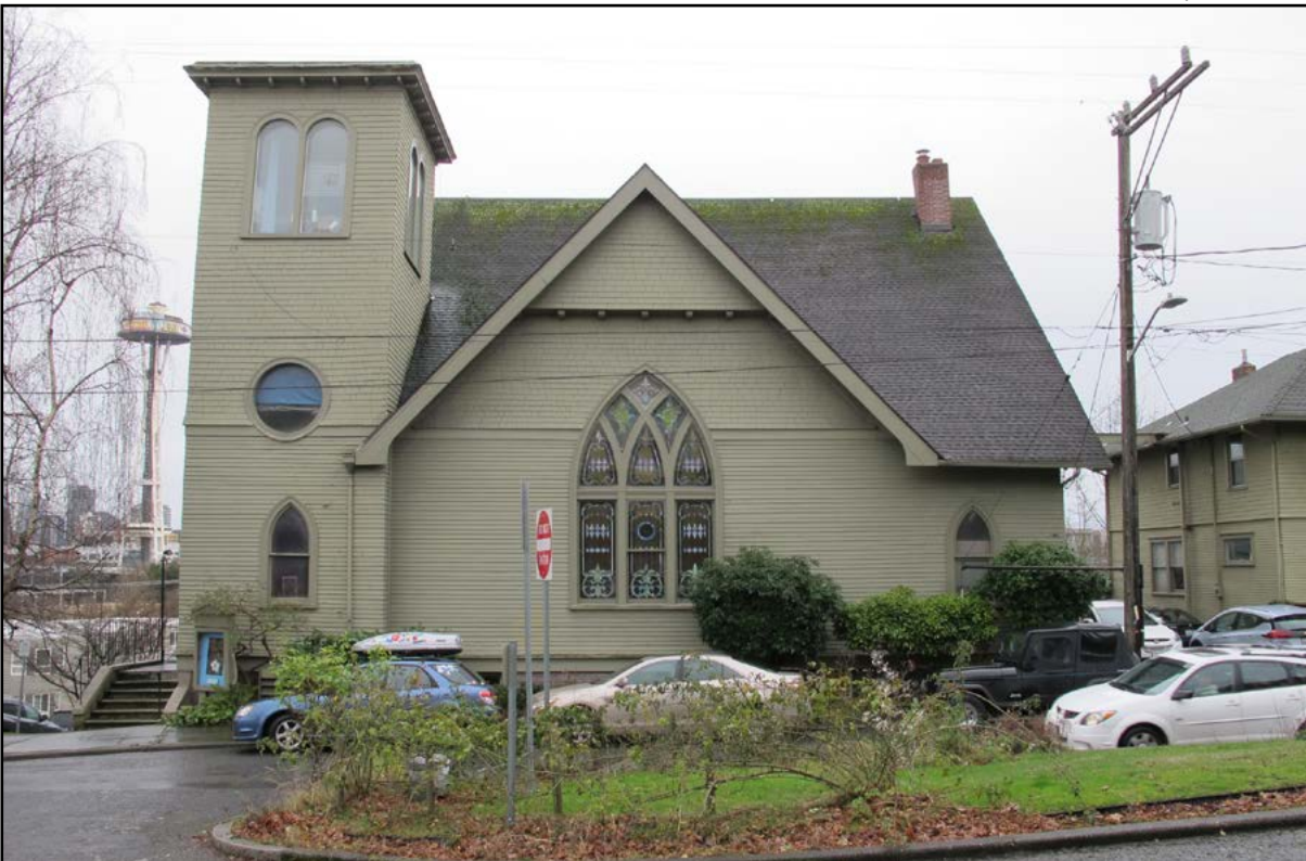
Figure 15 • Former church building, northern façade
