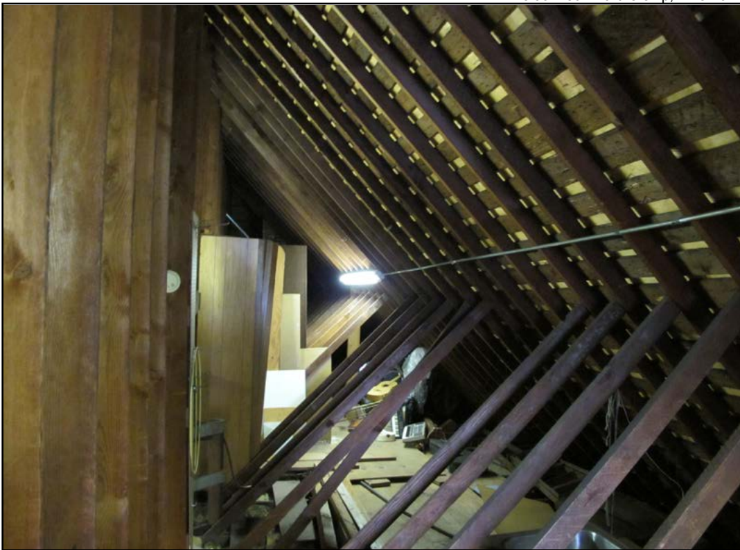
Figure 29 • Former church building, attic, main mass
