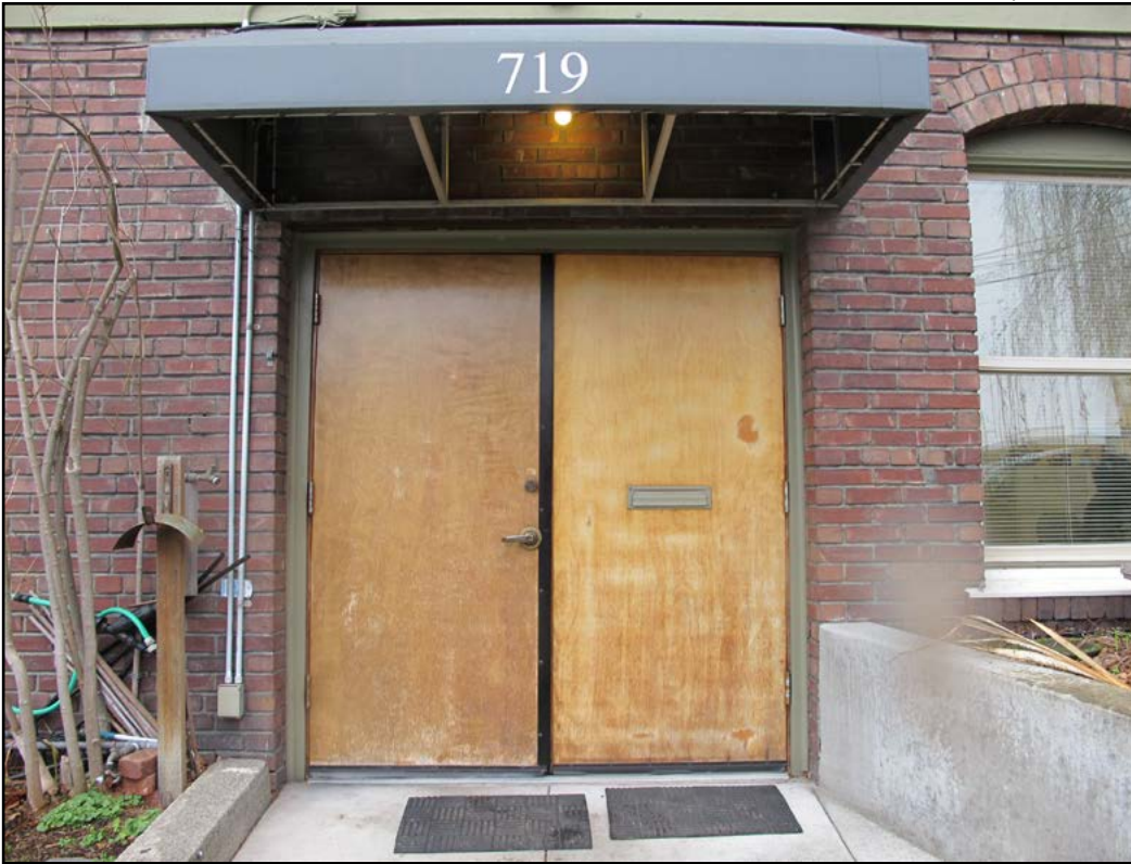
Figure 14 • Former church building, entry at basement level
