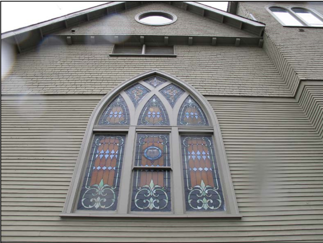
Figure 12 • Former church building, windows on eastern façade
